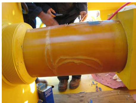
FIGURE 3. INSTALLATION ON THE MEASUREMENT STATION.
